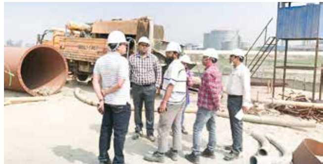
Lenders from Islamic Corporation for the Development of the Private Sector (ICD), Infrastructure Development Company Limited (IDCOL) and Lenders' Technical Advisors (LTA) from L&T-Sargent & Lundy Limited, India visited Gazipur plants.
