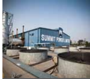
MADHABDI POWER PLANT | 35.30 MW
