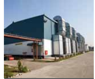
MADANGANJ POWER PLANT | 102 MW
