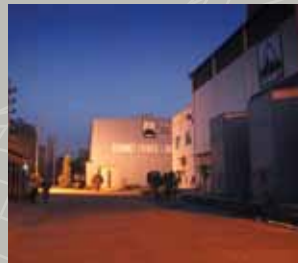
ASHULIA POWER PLANT | 44.75 MW
