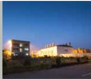
JANGALIA POWER PLANT | 33 MW
