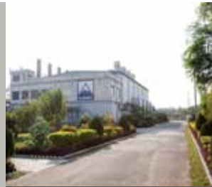
MAONA POWER PLANT | 33 MW
