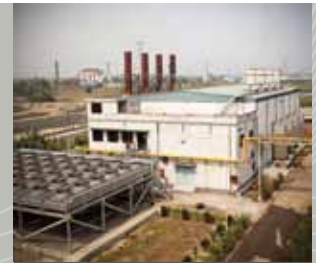
RUPGANJ POWER PLANT | 33 MW
