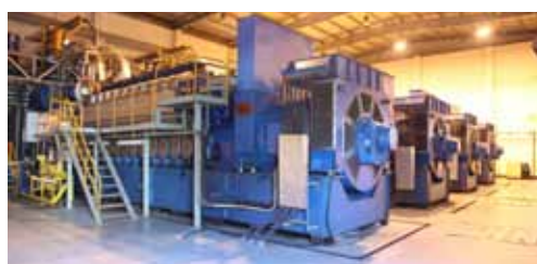
Maona Power plant (engine room)
