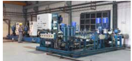
Madanganj Power plant
