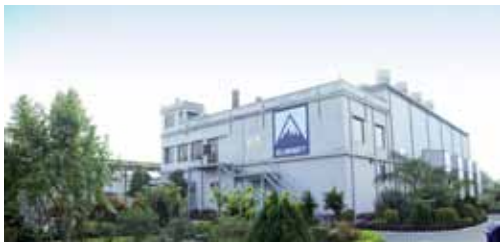
Maona Power plant
