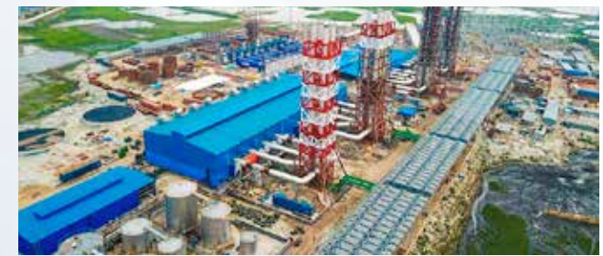
Summit Gazipur II Power Ltd –a 300 MW capacity power plant was completed in record time.
